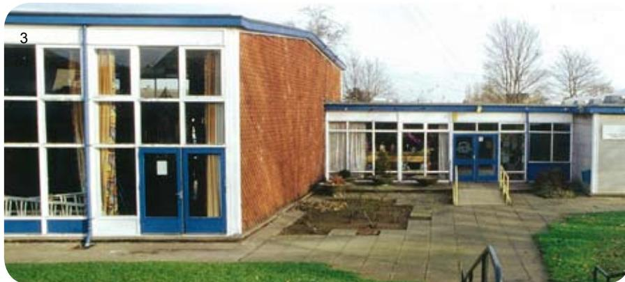
systemised school building comprising a lightweight steel frame system clad with variations of timber, tile hanging, curtain-walling and concrete panels.
