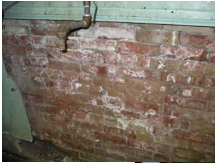
Interior Masonry Conditions
